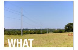
The Clendenin – Walton Area Improvements Project consists of building approximately 25 miles of new transmission line using steel H-Frame structures, three new substations and upgrading existing transmission facilities. The project will provide a robust transmission grid for customers in Kanawha and Roane counties.
